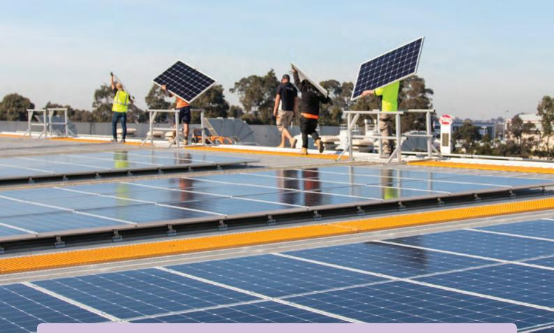
In November 2017, we installed a 2.1 MW solar array at our Sydney Parcel Facility, making it at the time, Australia's largest commercial solar system.
