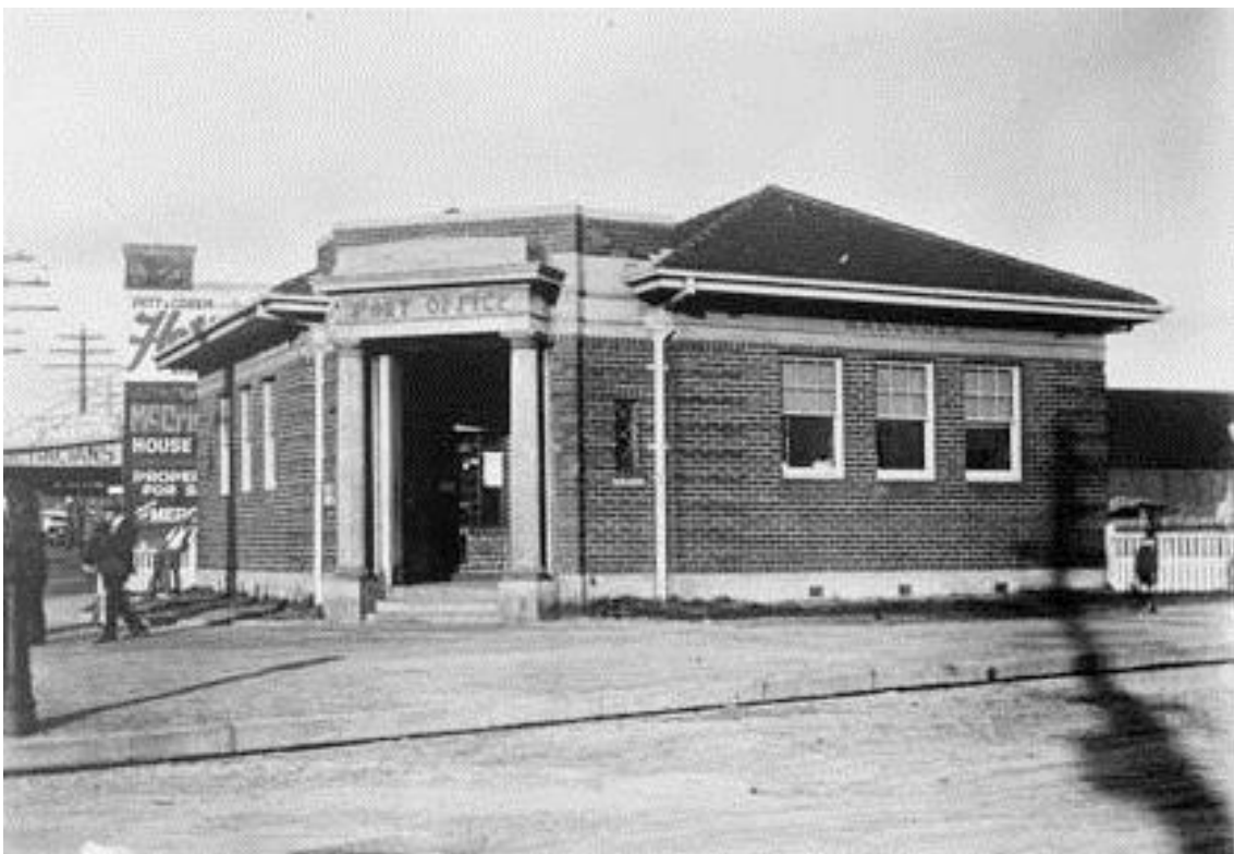
Figure 55 Mascot Airport Post Office, c. 1938 Source: National Archives of Australia, image no C4076, HN1445
