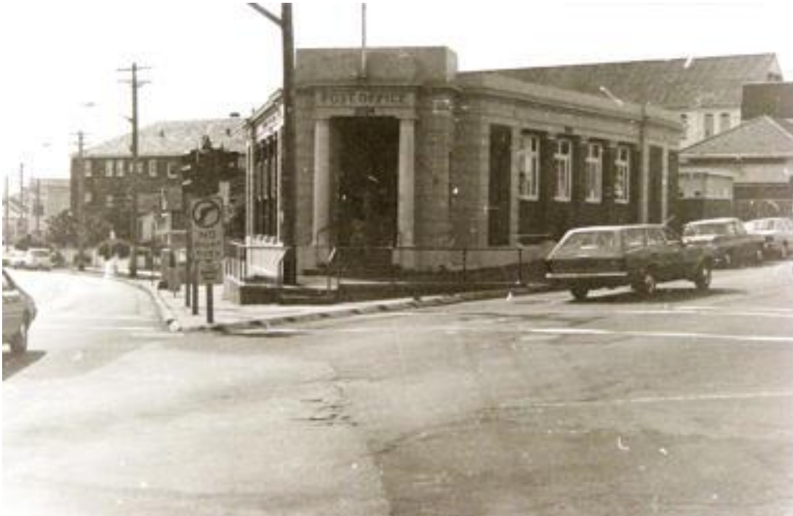
Figure 56 Charing Cross Post Office, built 1923, corner of Bronte Road and Carrington Road, Waverley, 1975 [also referred to as Waverley Post Office] Source: Waverley Council Image Library
