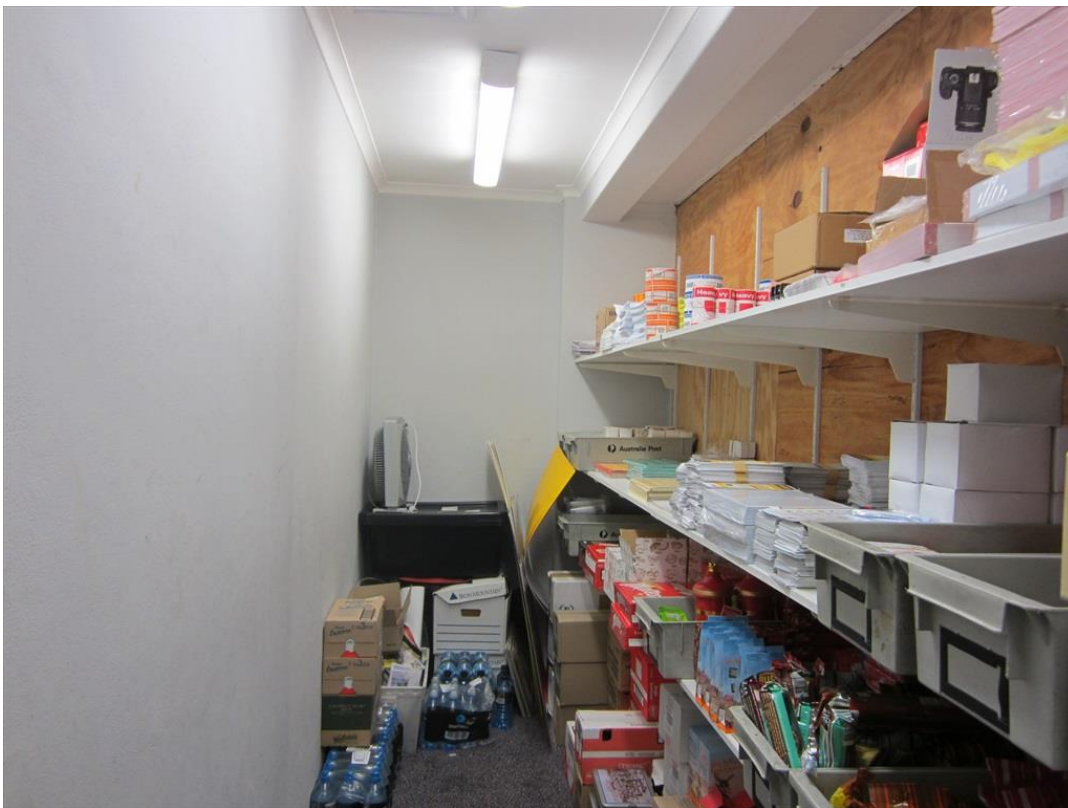
Figure 47 Store space to the west of the porch originally occupied by the phone booths; the ceiling beam indicates the line of the original opening
