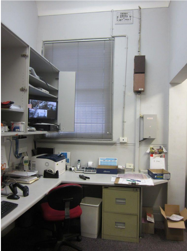
Figure 48 West wall of office space to the south of the porch; note remnant sill, wall vent and inscribed bead at sill height
