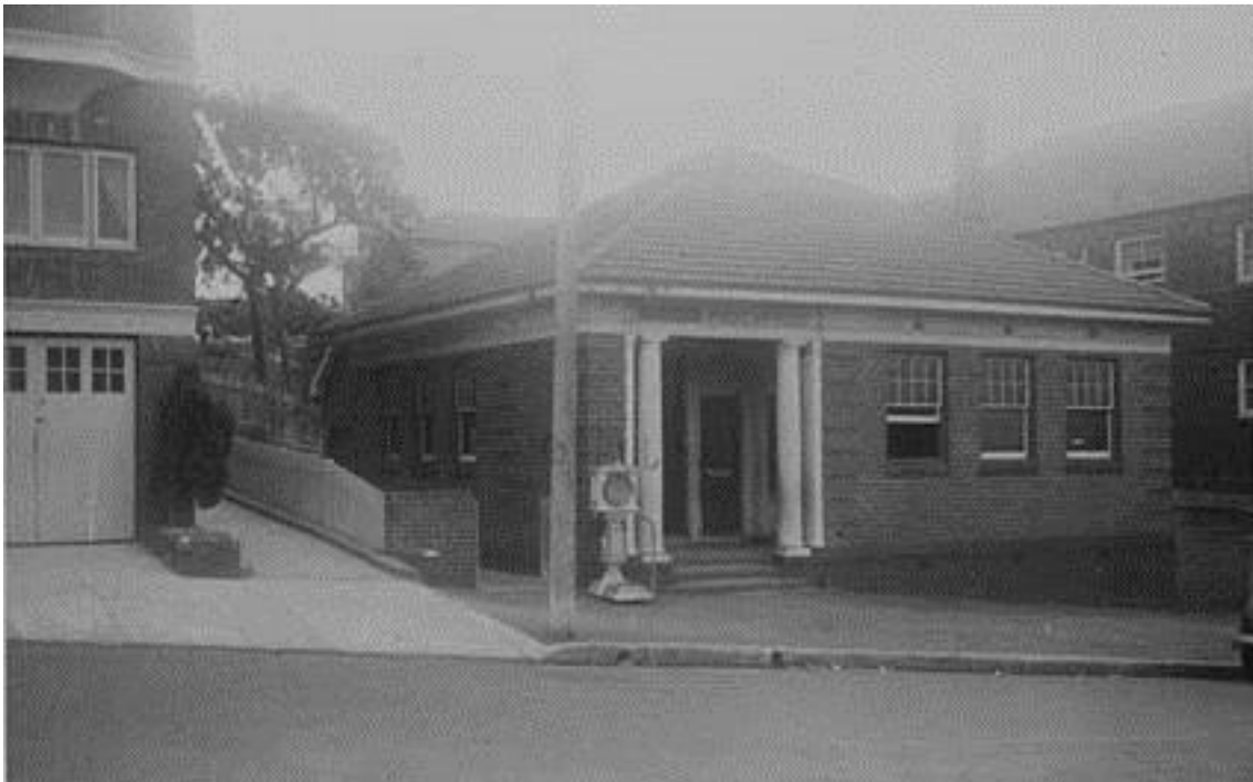
Figure 58 Coogee Post Office, 1946 Source: National Archives of Australia, image No C4076, HN 17066
