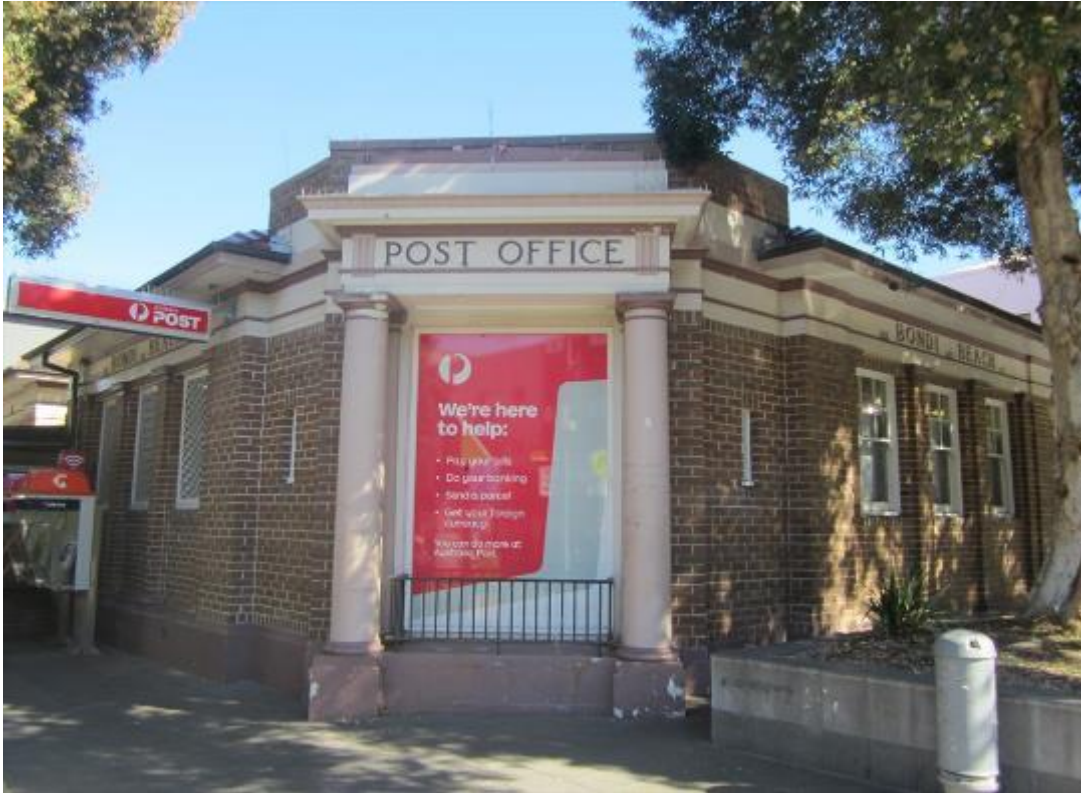
Figure 33 North-east corner entry to the Bondi Beach Post Office; note the infilling of the original entrance and steps
