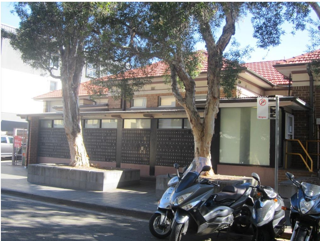
Figure 38 Hipped roof pavilion, post office boxes and works space additions to the south of the c. 1922 post office
