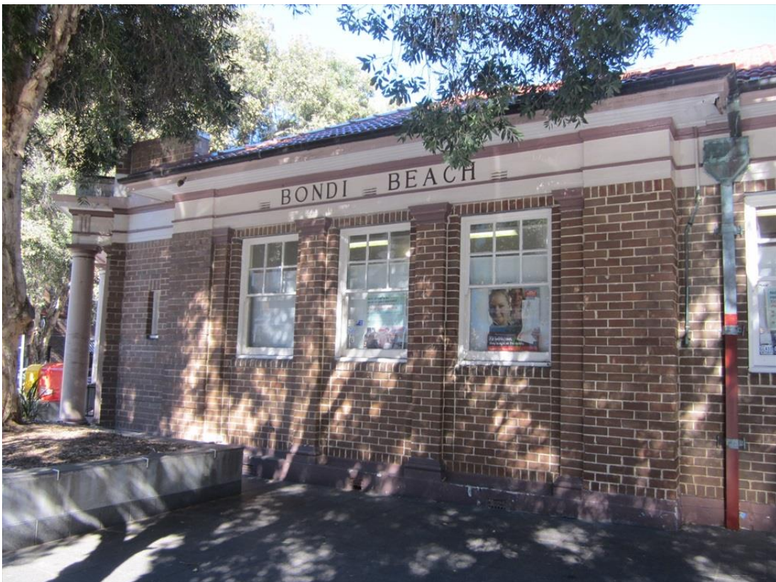
Figure 34 North façade of the c. 1922 post office to Hall Street; internal shop fittings are visible through the windows
