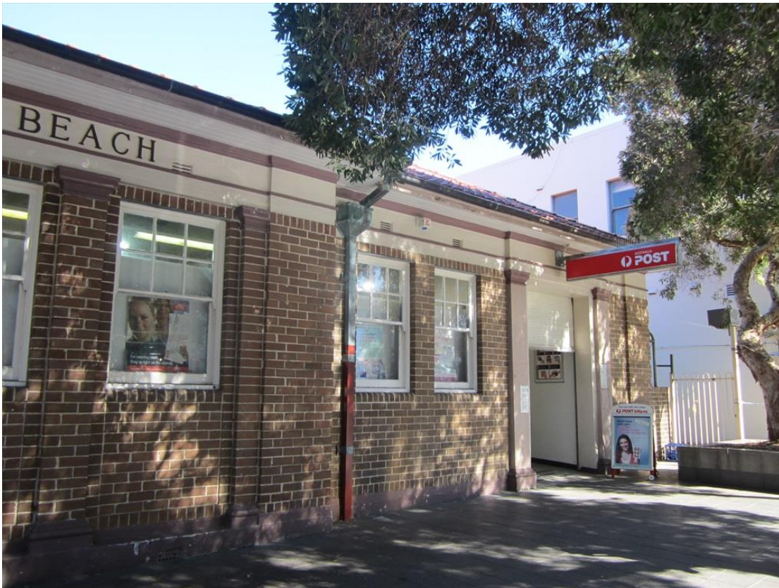
Figure 35 Western addition and entry to the post office on Hall Street, constructed in c. 1934
