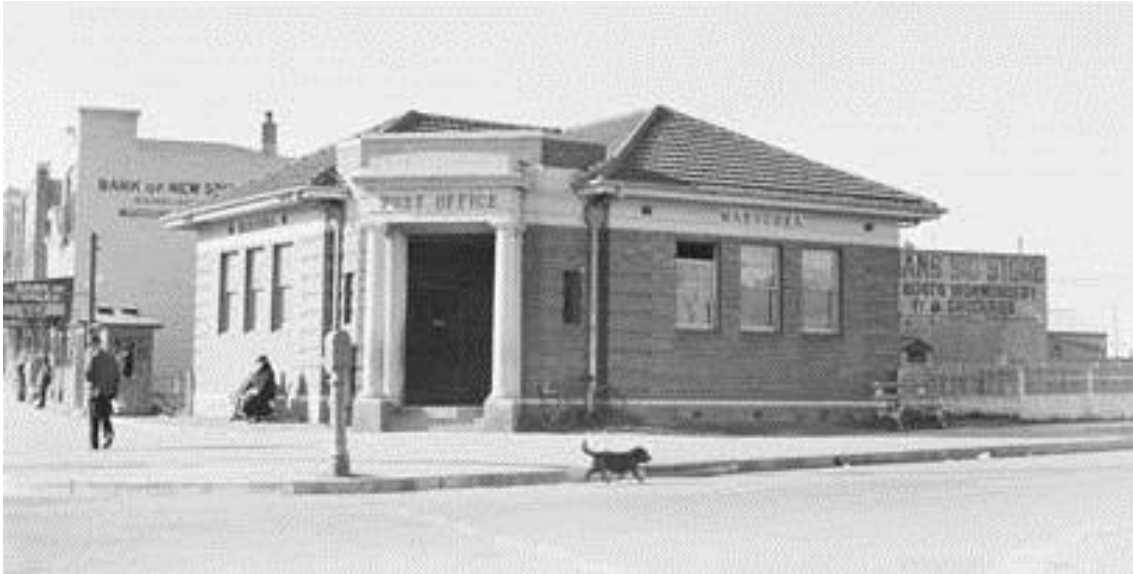
Figure 13 Maroubra Post Office in 1947 Source: National Archives of Australia, image no C4078, N2982
