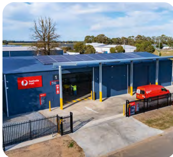
The new Australia Post facility in Corowa, New South Wales.
