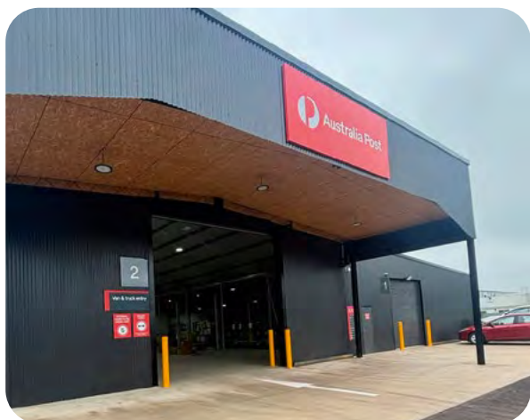
The new Australia Post Parcel Facility in Benalla, Victoria.
