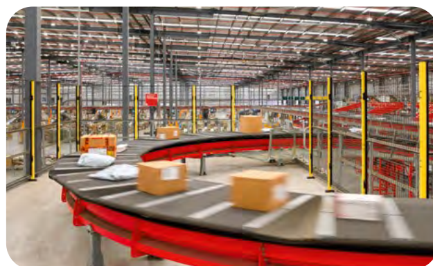
Processing equipment is used to reduce manual handling and injury risks.
